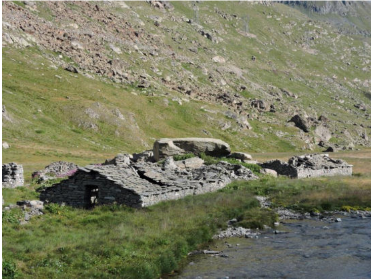
Abandoned alpage building, Aosta Valley.
